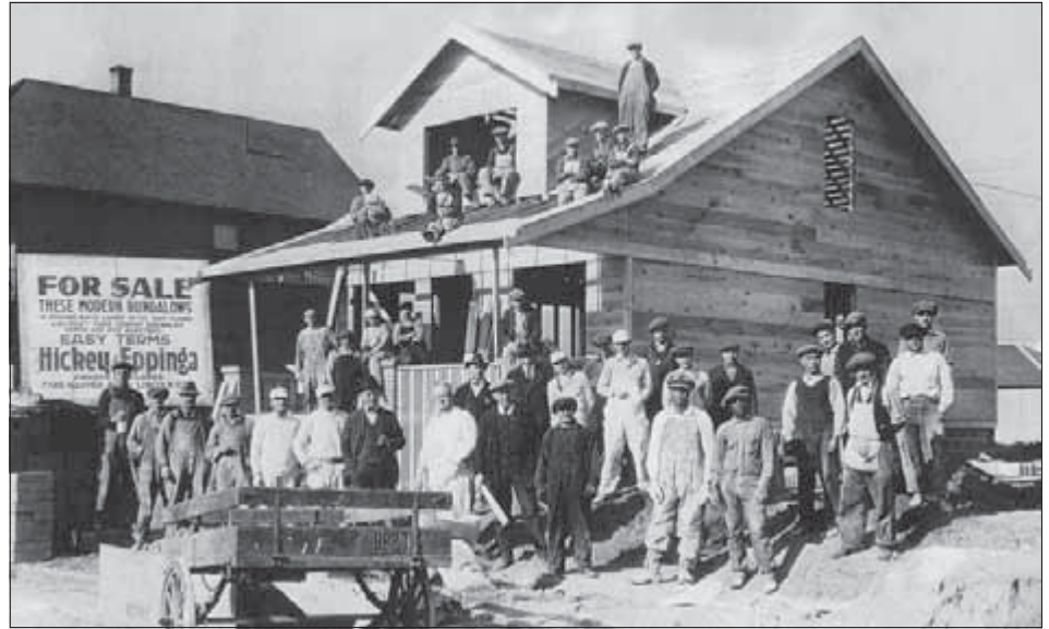
A number of the male members of First Detroit CRC were skilled craftsmen who built residential subdivisions on Detroit's east side. This bungalow was being built by the firm of Hickey and Eppinga, who also were members of the congregation. Photo courtesy of Rev. Jacob Epping, son of Dirk Eppinga, one-half of the home building partnership.
