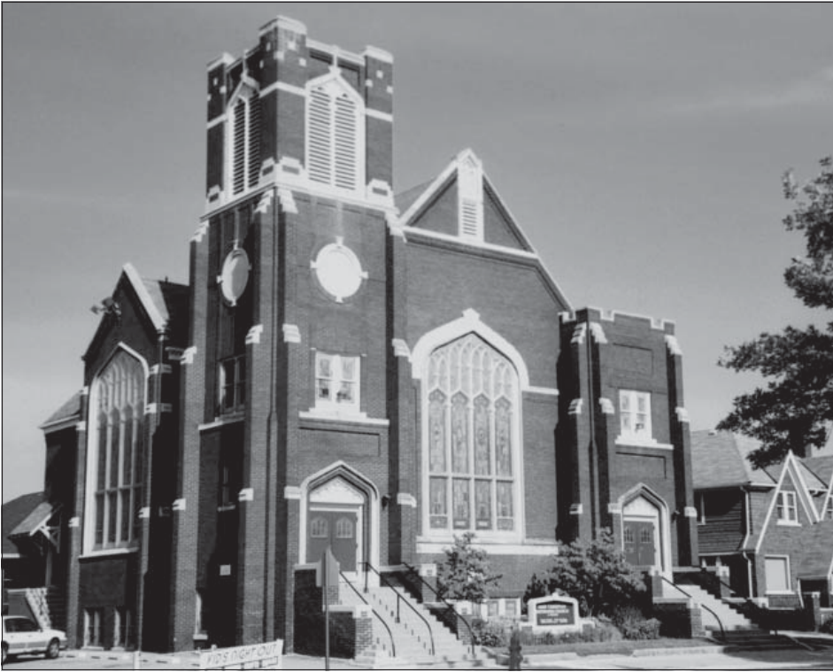
On 5 February 1925 the congregation dedicated its new structure at 1444 Maryland Street. Although most of the new Christian Reformed churches in West Michigan were designed by J. & G. Daverman, the Detroit congregation wanted an edifice that did not have a “certain sameness of style” of the West Michigan buildings. Photo courtesy of James Evenhuis.
