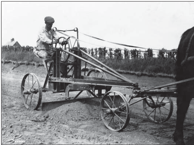
A horse-drawn grader similar to the one Hoekstra used for sidewalk work in the Chicago area. Image courtesy of Bass Photo Co. Collection, Indiana Historical Society.
