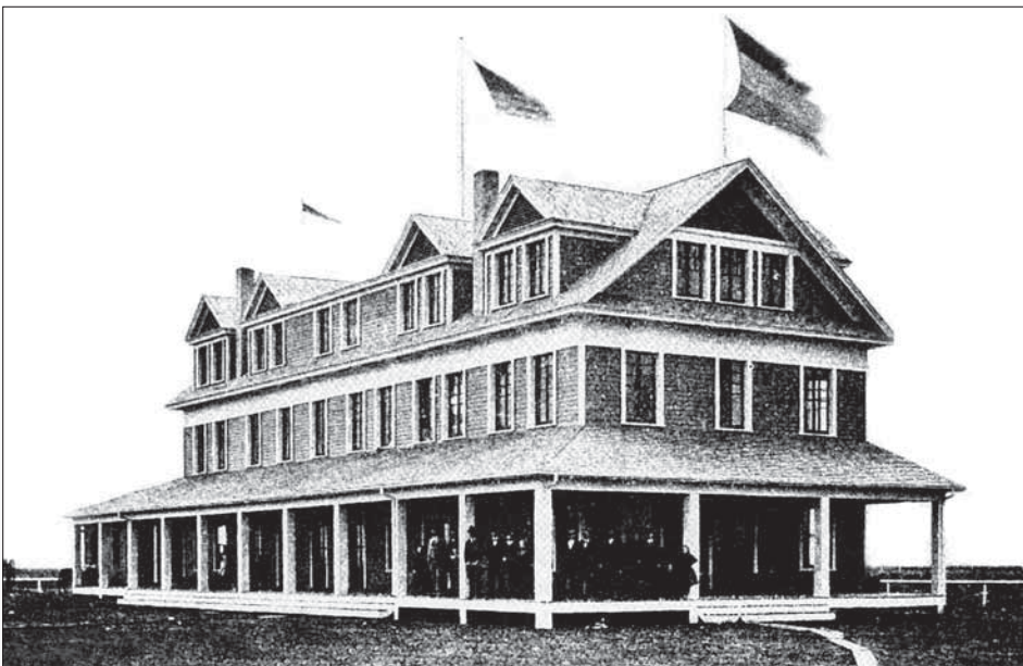
The Orange Hotel. Bricks for the foundation, 80-foot well, and chimneys were handmade. Image courtesy of the Nederland Historical Society.
