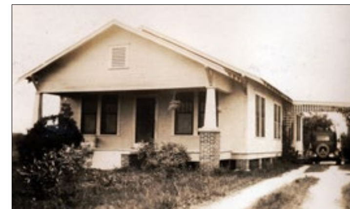
The Renkema house in Texas; note that it is built off the ground. Image from the collections in Heritage Hall, Calvin College, Grand Rapids, Michigan.
