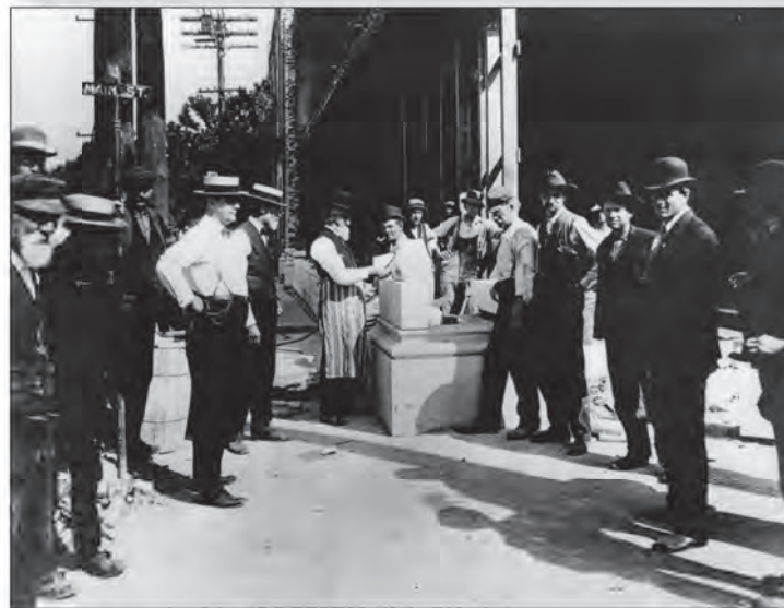
Laying the cornerstone at the Zeeland State Bank, 101 E. Main Street, ca. 1909. Jacob Den Herder at the stone. Courtesy of the Zeeland Historical Society.
