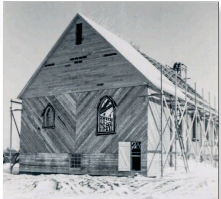
Barrie Christian Reformed Church under construction.
