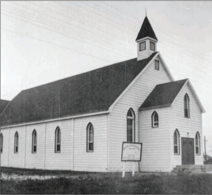
Wellandport Christian Reformed Church.
