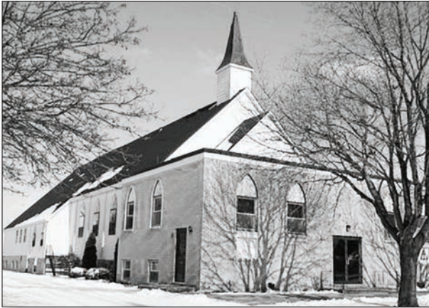
Wyoming CRC, with an addition on the back.
